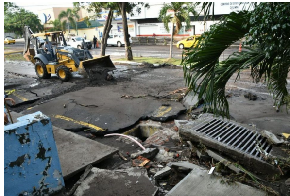
Figure 4: Damage caused to 20 de noviembre Avenue by the overflow of Manrique brook. (Source: El Diario de Colima newspaper, August 3, 2018)
